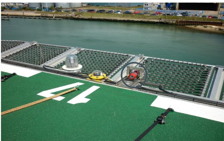
Figure 4 Micropack FDS301 Helideck Installation
