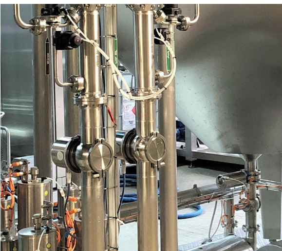
Figure 1: Yeast propagation plant
