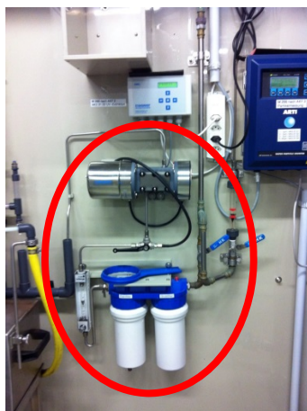
Pict. 5: ColorPlus bypass in raw water with sample filtration
