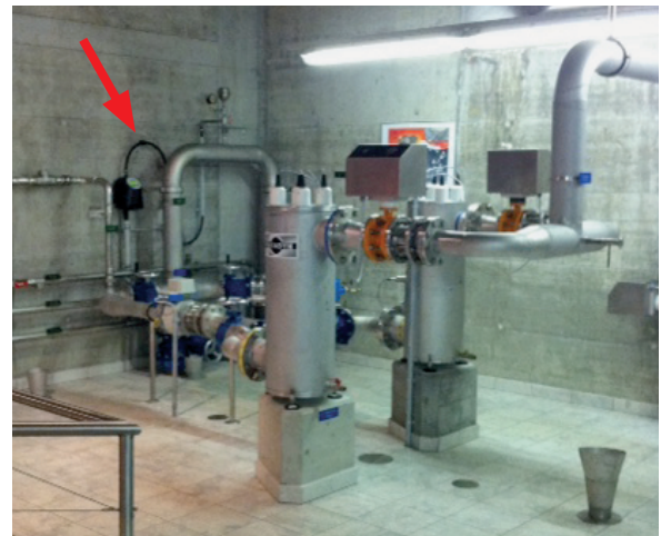
UV reactors with AquaScat WTM before/after disinfection
