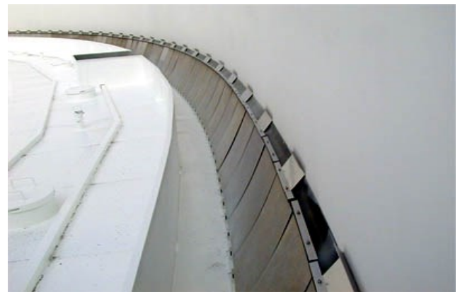
Typical rim seal and foam dam.
