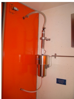
Picture: VisGuard Mini-extractive installed in an SOS-niche
